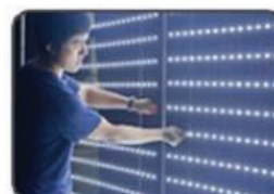
Safety Voltage in 12V
